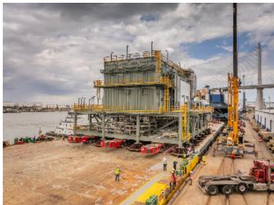
CAPTION: dteq's engineered solution for the safe and efficient transfer and securing of a 25,778 CBM LNG module from a barge to a deck carrier.
