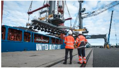
CAPTION: dteq providing personal on-site supervision of port crane loading operations.
